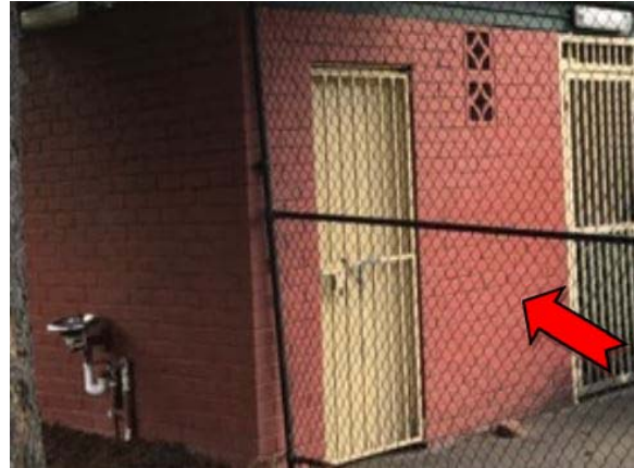
Photo 2. Exterior, throughout, walls – suspected lead-containing red upper paint system.
