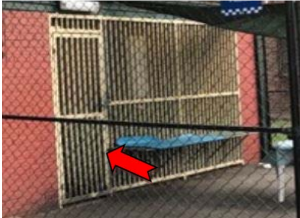
Photo 1. Exterior, throughout, doors and door frames – suspected lead-containing yellow upper paint system.
